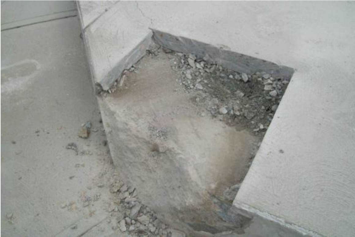
TEST CUT #2 NEAR THE ACCESS RAMP, REVEALED A Poured CONCRETE WALL
